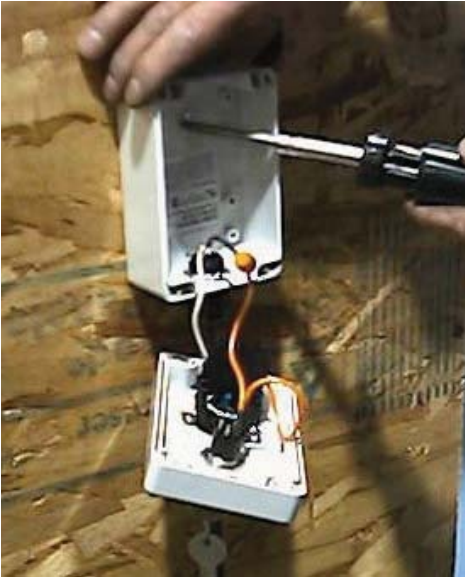
FIG. 17- MOUNT LOWER CALL STATION
