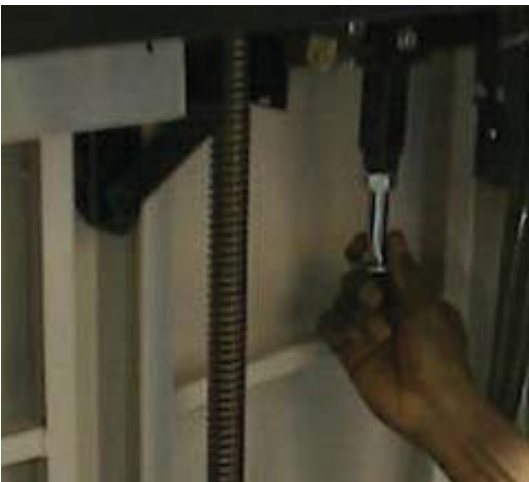
FIG. 4- INSTALLING LOWER MECHANICAL STOPS
