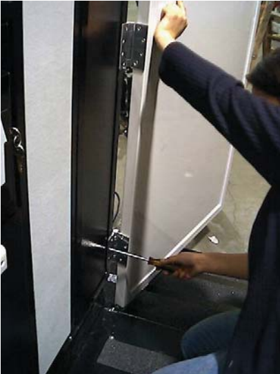
FIG. 8- MOUNTING GATE TO CONTROL WALL EXTENSION
