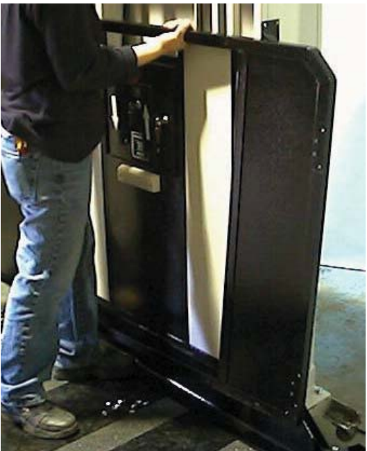
FIG. 5A- INSTALLING CONTROL WALL EXTENSION
